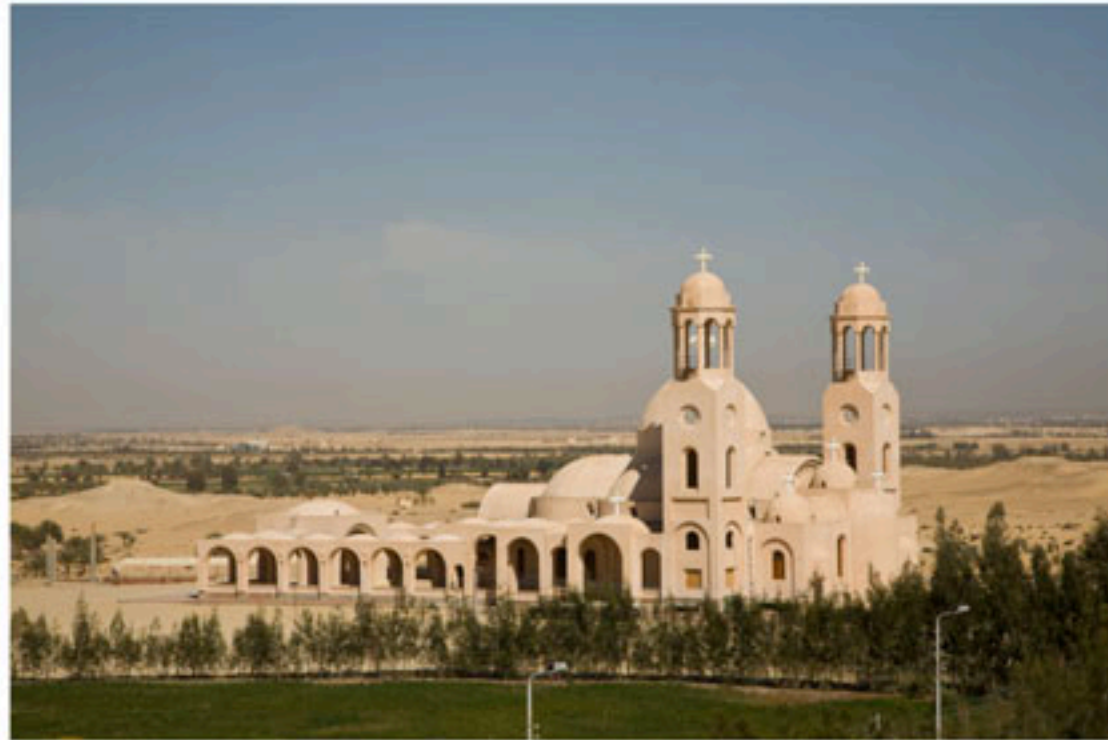
Above Left: south altar screen of Cathedral. Above Right: view toward north from south altar of Cathedral. Below: Cathedral exterior (see map page 3).
