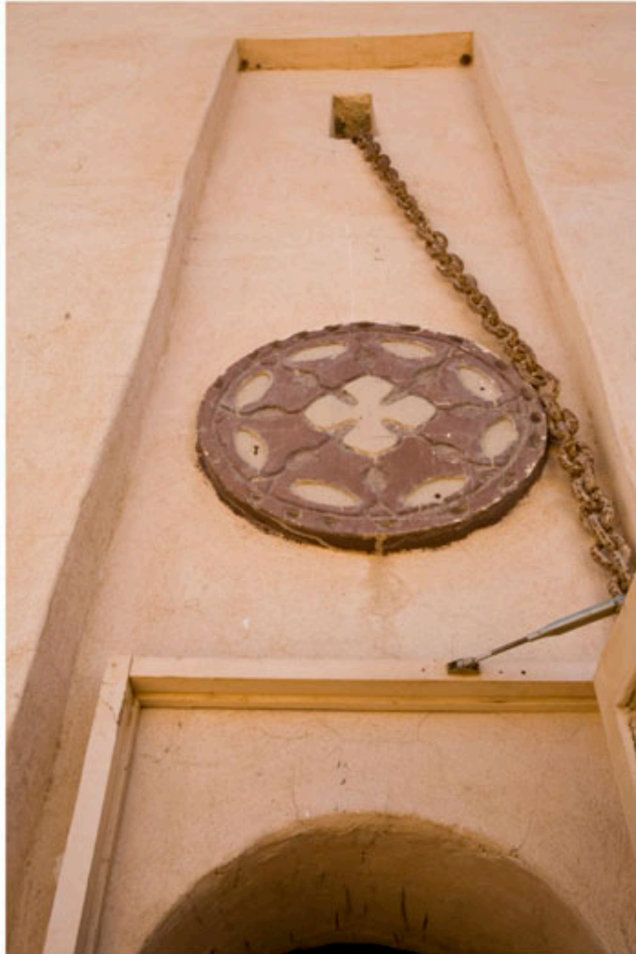
Detail above door to keep, upper drawbridge (Area A).
